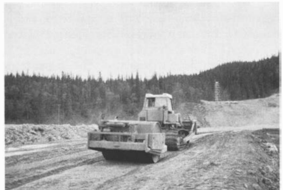
Fig. 5. Compaction of till for an earth-dam core by a vibratory roller.
