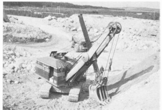
Fig. 2. Excavation of till with power shovel.
