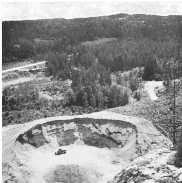
Fig. 38. Excavation in the plain at 139 m a.s.l., SW. of Kättestorp (cf. Fig. 39). Photograph taken June 1971.
